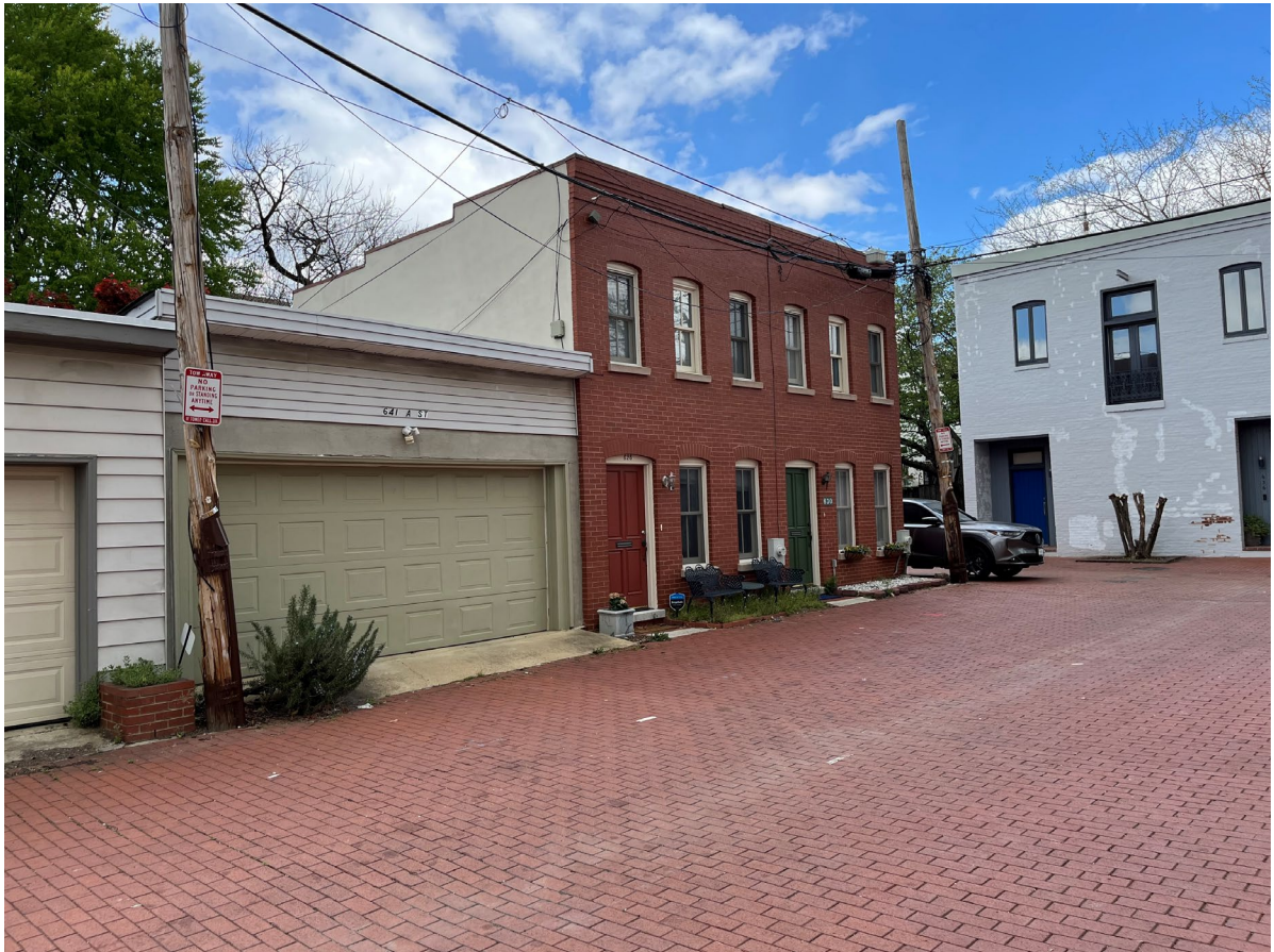
ALLEY, LOOKING EAST
