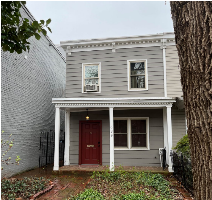
EXISTING FRONT FACADE
