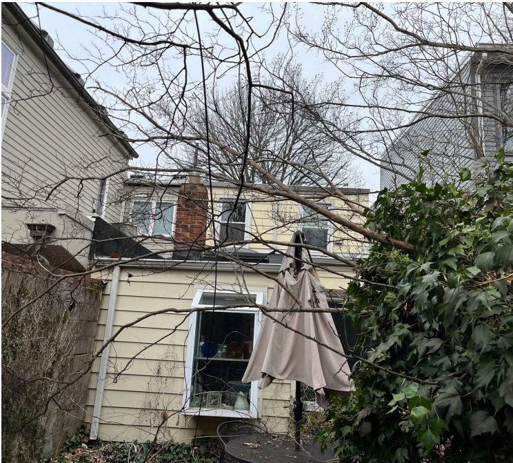
EXISTING REAR FACADE
